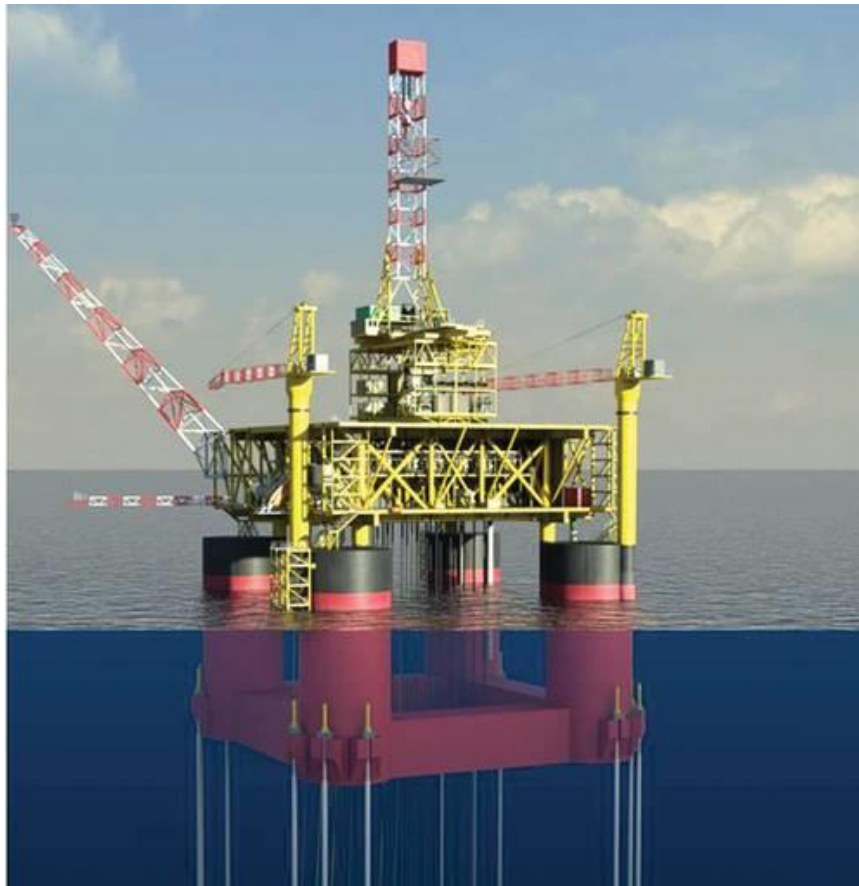
Figure 1 Tension Leg Platform (TLP) used for deep-water offshore operations.
